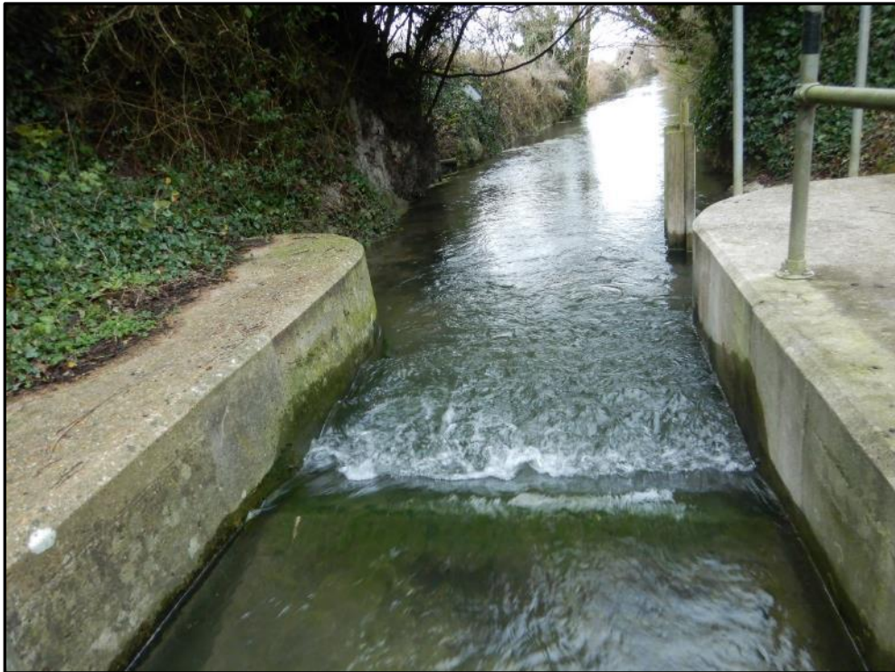
Pic 35 – The EA gauging station, a barrier to the upstream movement of small fish but adult trout would be able to traverse it (TL 60873 69589).
