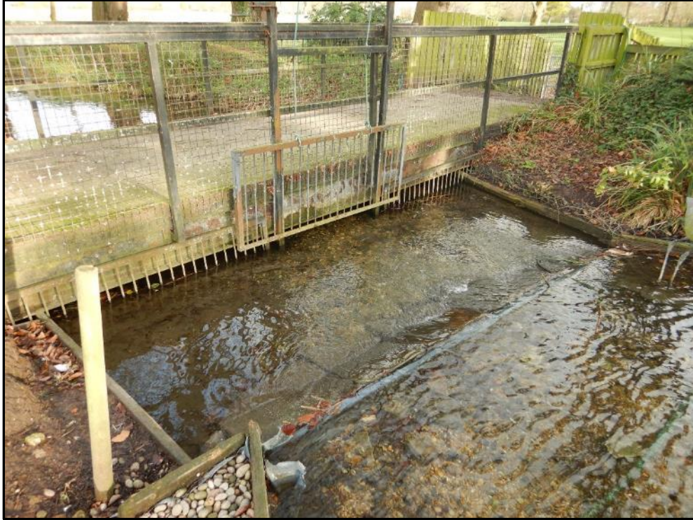
Pic 20 – The weir within the Regal Lodge grounds is used to retain water for a wildfowl collection. It is degrading the river.
