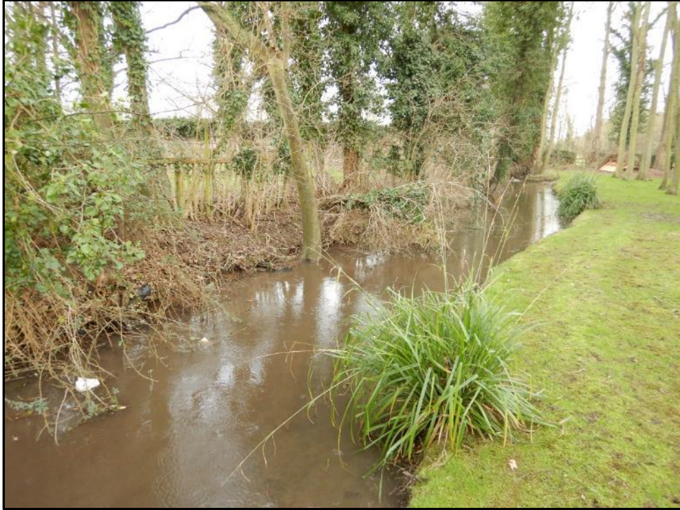
Pic 24 – The side-channel around the mill, it is also impounded and full of silt.
