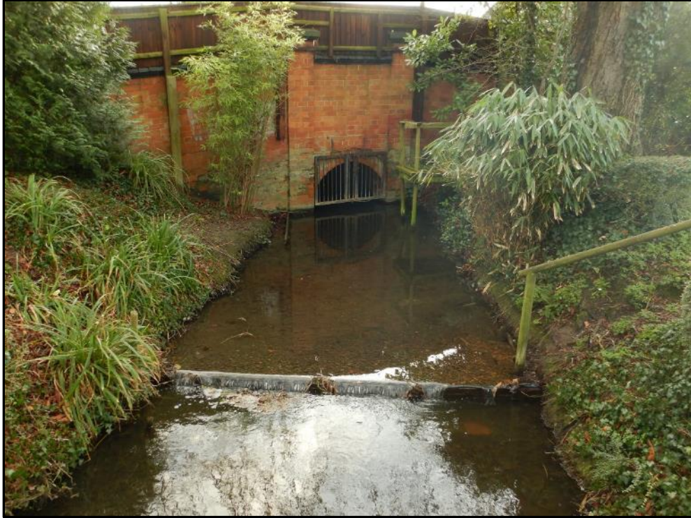
Pic 19 – This weir is affecting the river for at least 150m upstream to New River Green. It should be removed as it provides no benefit to the property in which it is located.
