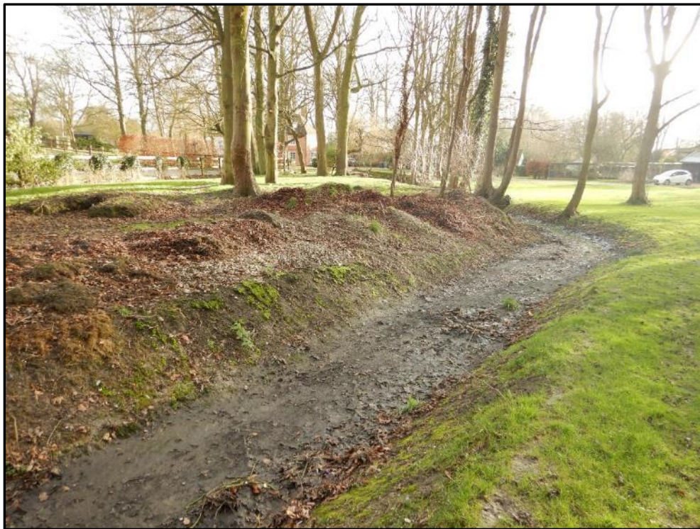
Pic 26 – The dry river channel emerging from the mill. The channel has clearly conveyed water in recent times, however the dark colouration is suggestive of road run-off. Note the large volume of leaves dumped on the bank top and slopes.
