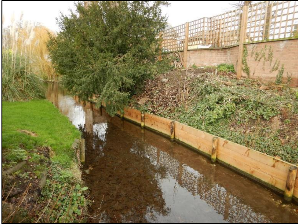
Pic 13 – The river after Church Lane, the channel is devoid of any plants, the left bank is supported by gabions and the right bank by new toe-boards. Both means of bank stabilisation degrade the river.
