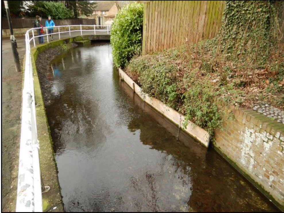
Pic 11 – The river in Church Lane had no habitat to sustain trout nor water voles. Note the recently installed toe-boards.
