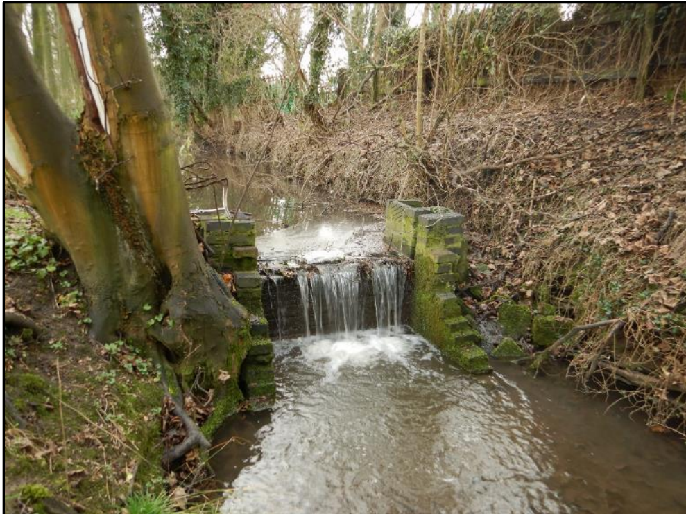
Pic 25 – A partially defunct structure that impounds the reach above it should be removed.
