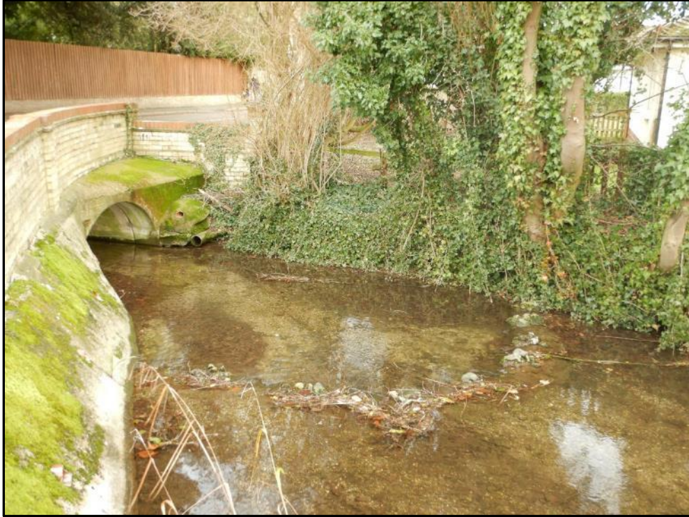
Pic 9 – The road bridge of Ducks Lane holds water back within the pond, and a concrete and stone weir has been constructed to retain a greater head of water.
