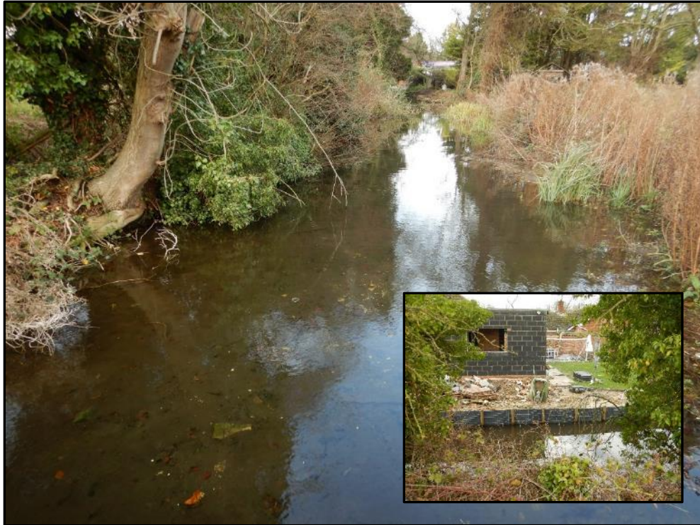
Pic 5 – The river downstream of the A14 is overwide and impounded. Where gardens back-on to the river hard bank revetments are the usual inappropriate means of bank treatment.
