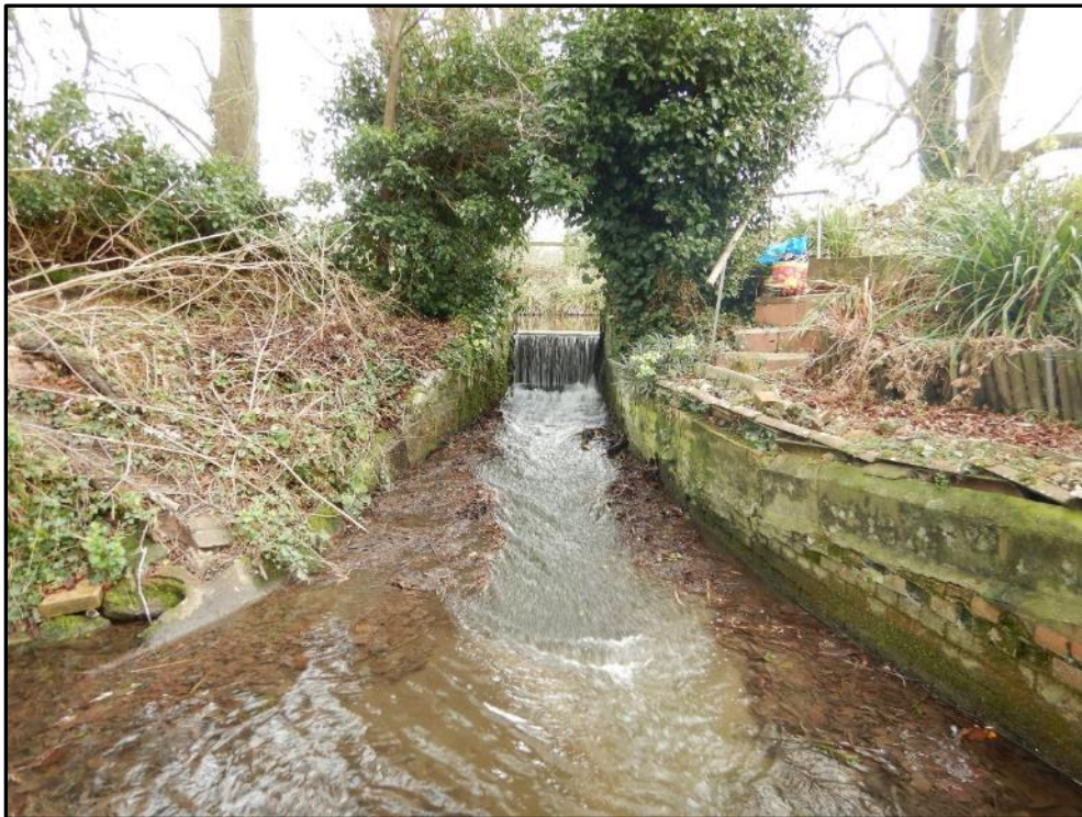
Pic 22 – The side-sluiice now conveys the entire river flow.
