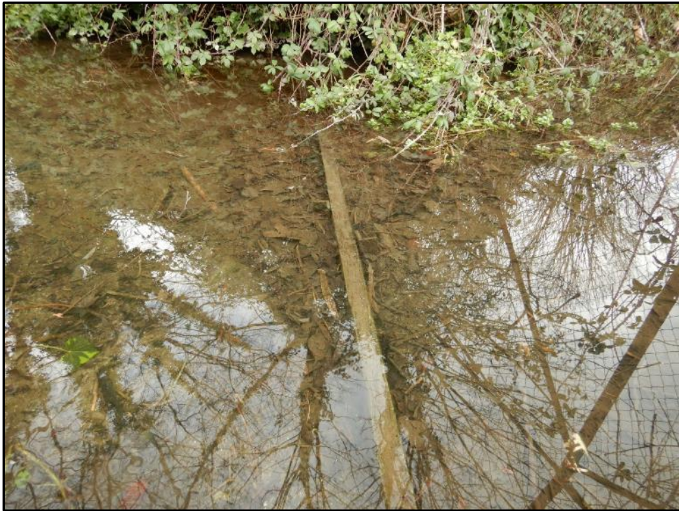
Pic 17 – The previous water-retaining board is now drowned-out by a further impoundment downstream.
