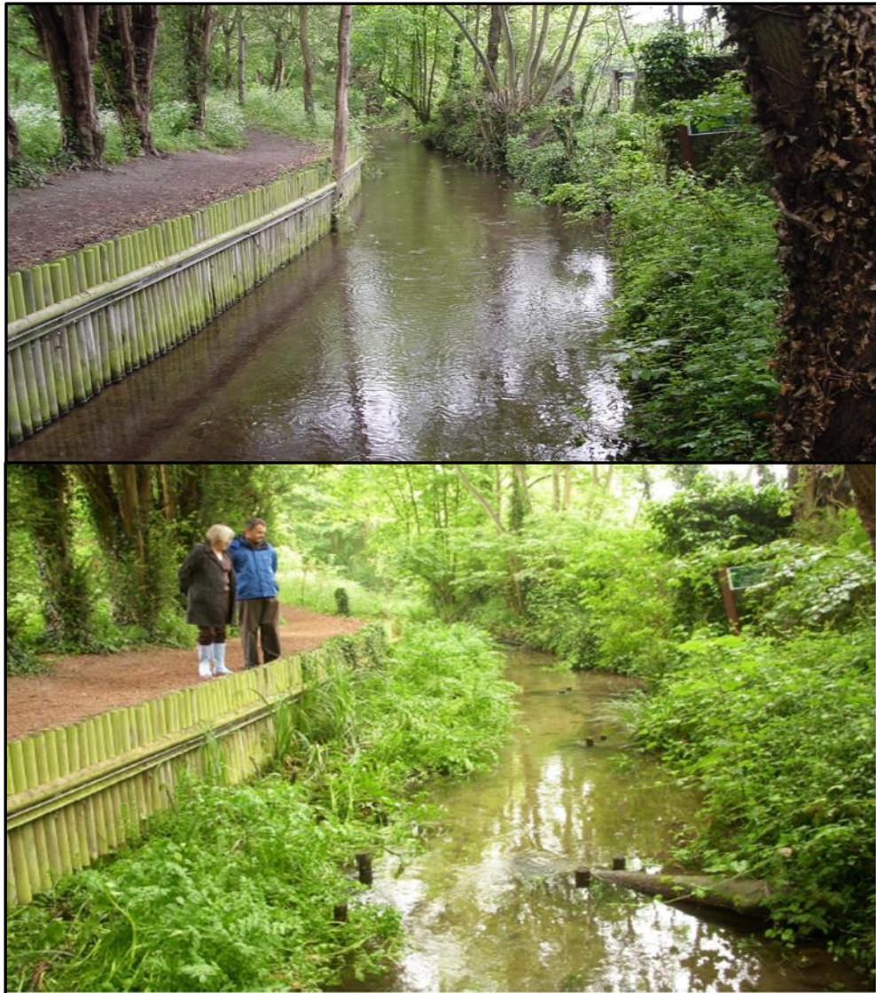
Pic 28 – The use of brushwood mattresses combined with pre-planted coir rolls enabled rapid marginal vegetation growth, which in turn provided water habitat and an important connection between existing populations.
